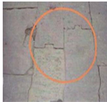
Fig. 20-Dowel joint
