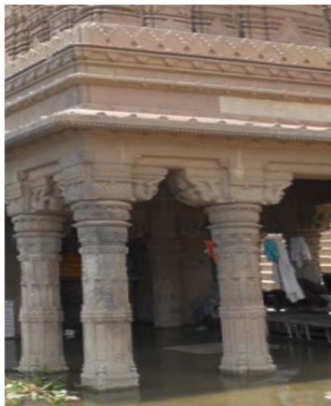
Fig. 12: Trabeated System
